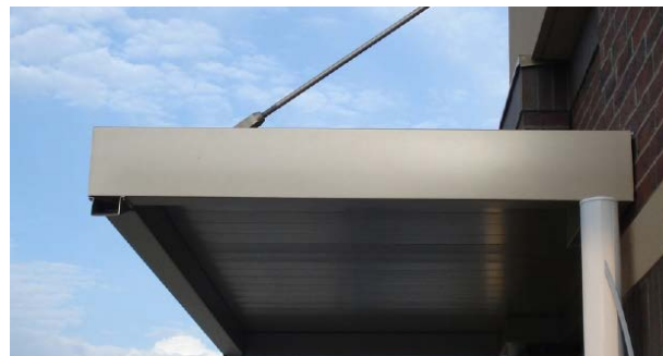
Metal Details and Brackets
