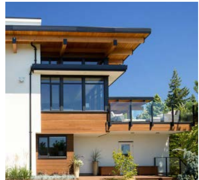
Exposed beams with modern downspouts & metal trim.
