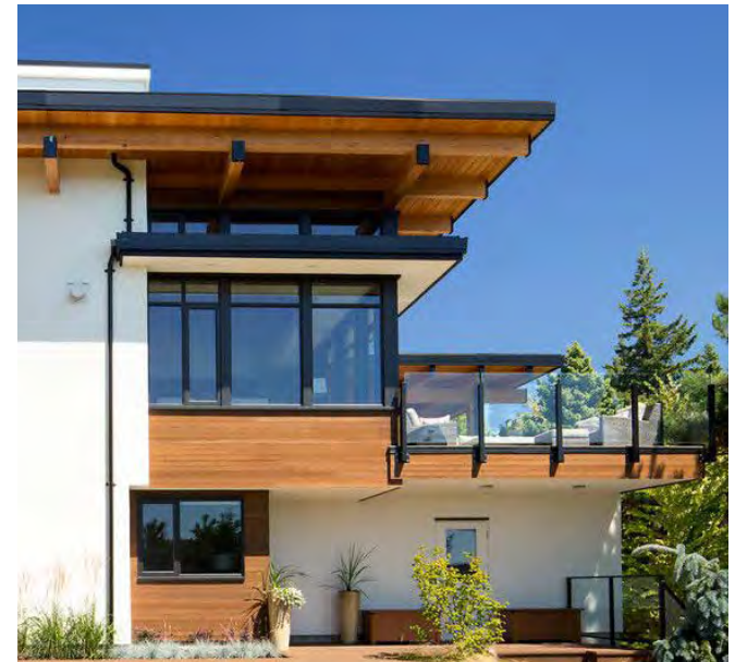
Exposed beams with modern downspouts & metal trim.
